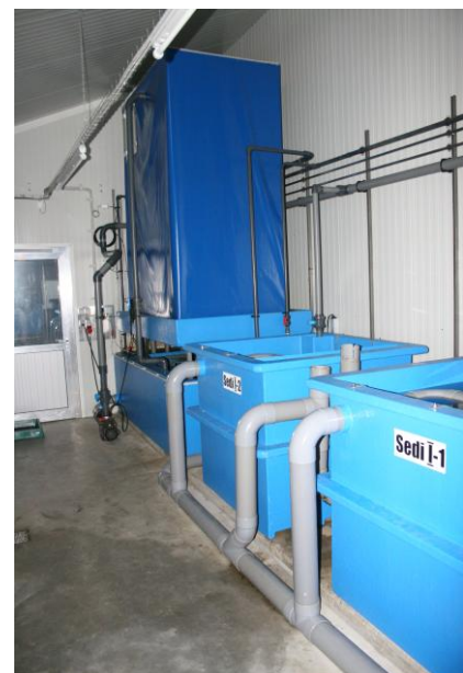
Figure 1. Recirculating aquaculture system (RAS) operated in the NEMATIC pilot facility at the FishGlassHouse (FGH), University of Rostock. The system consists of nine culture tanks (left) and a water treatment unit (right) including a sedimentation tank for mechanical filtration and a trickling filter for biological treatment.
